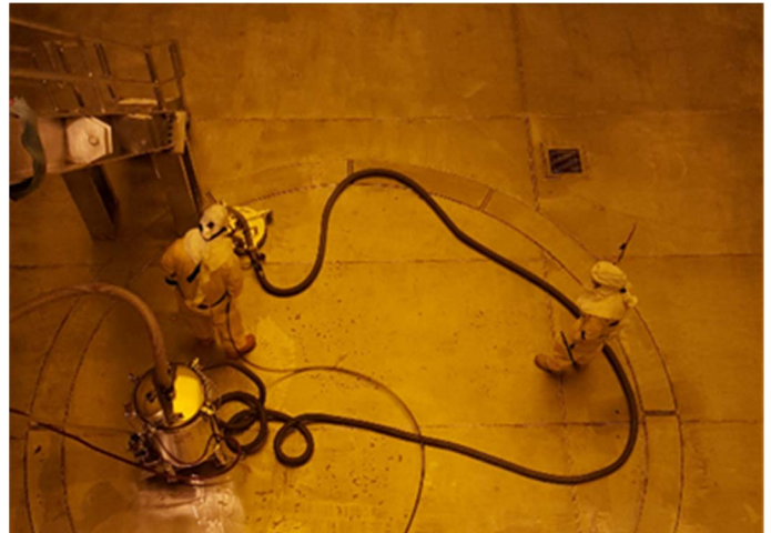
D-CAT™ Operation in BWR Dryer Separator Pit
