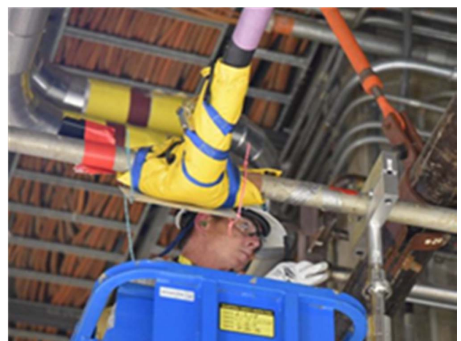
NU-DEC™ pipe decon application at US BWR
