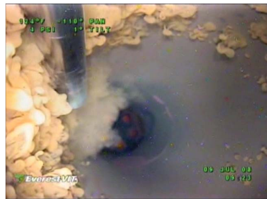
BWR jet pump cleaning
