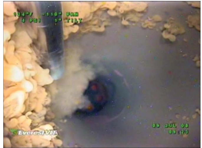
BWR ultrasonic jet pump cleaning
