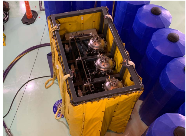
AMFM-S300 installation at BWR site
