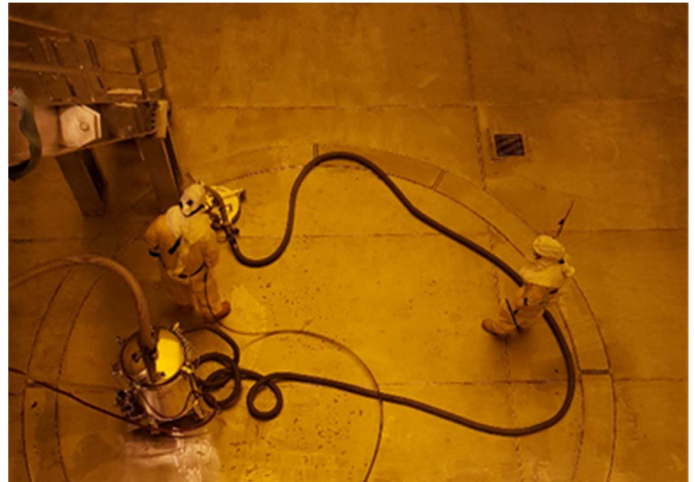
D-CAT™ Operation in BWR Dryer Separator Pit
