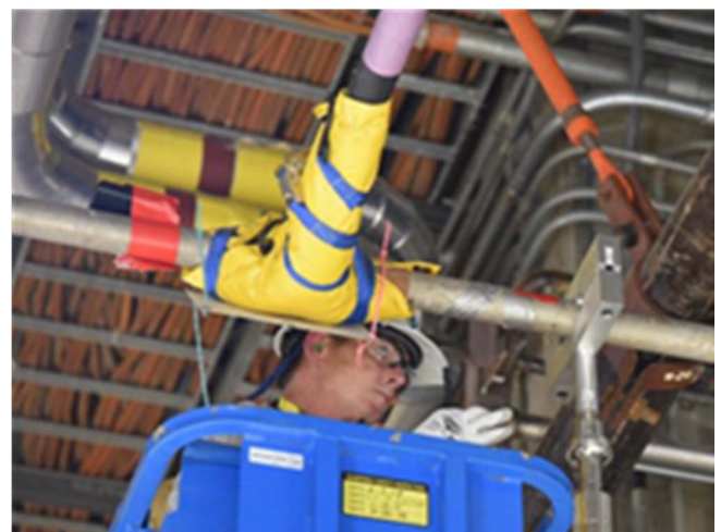
NU-DEC™ pipe decon application at US BWR
