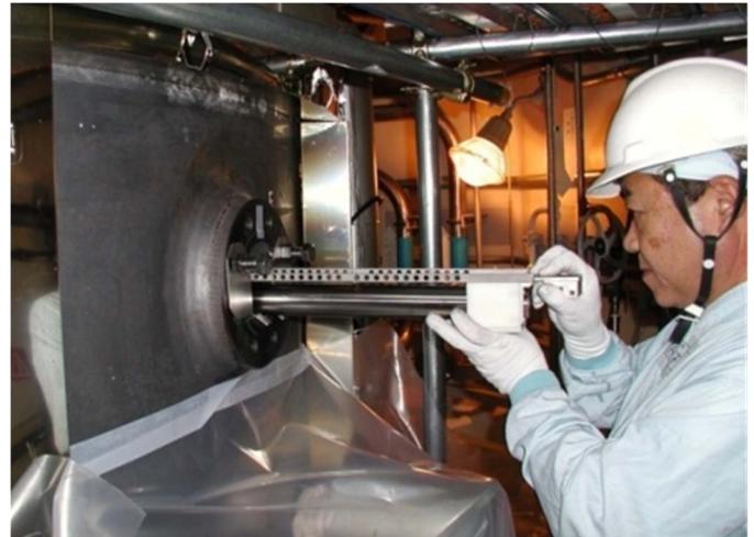
Insertion of ultrasonic transducers and delivery tooling into SG access port
